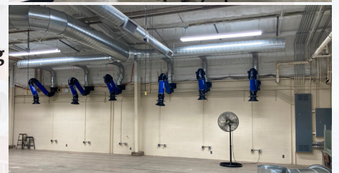
Top Photo: Newly renovated BAE Lab room 129. Bottom Photo: New welding lab. Photos by Dr. Mari Chinn
