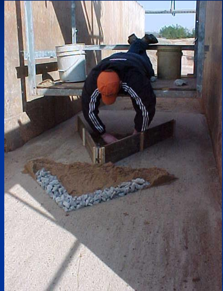
Prepare Structures Using Template
