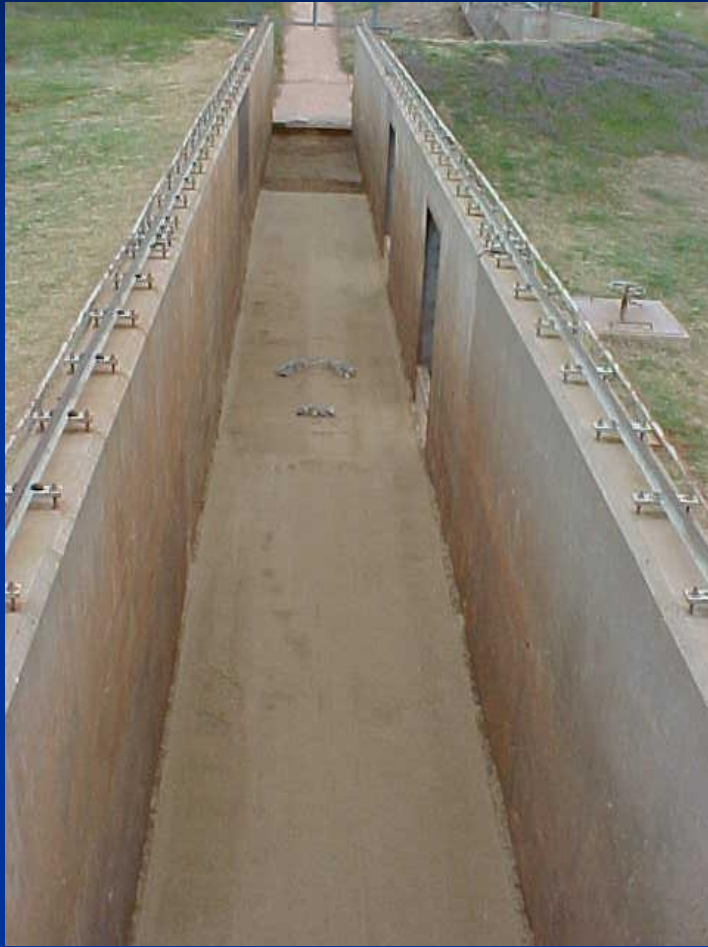
Prepare Level Bed
