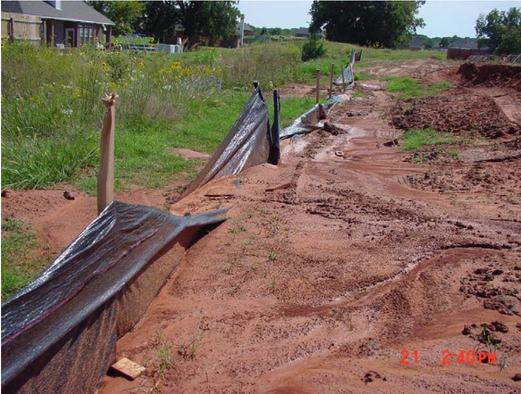
Figure 3. Failure resulting from Excessive Stretching and Overtopping (Barfield et al., 2000)
