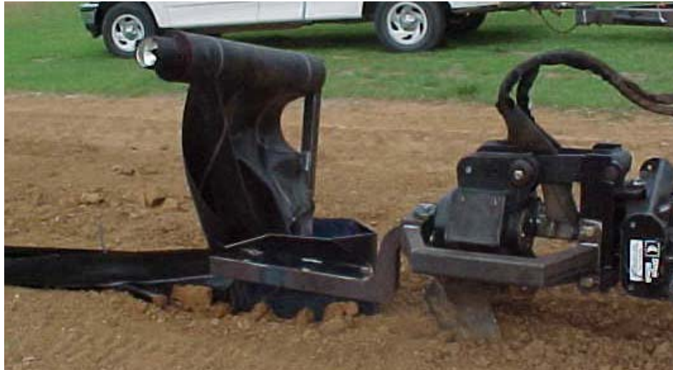
Figure 29. Fabric Unrolling due to Wind
