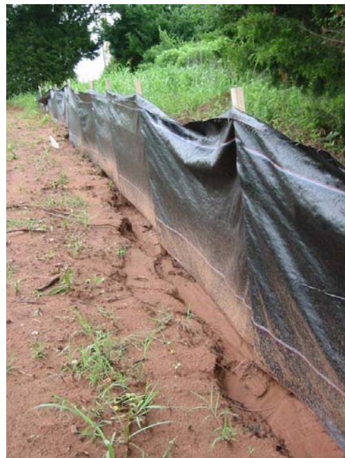
Figure 2. Failure due to concentrated parallel flow 2
