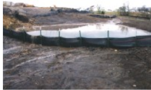
Figure 1. Properly Installed Silt Fence (Salix, 2000)
