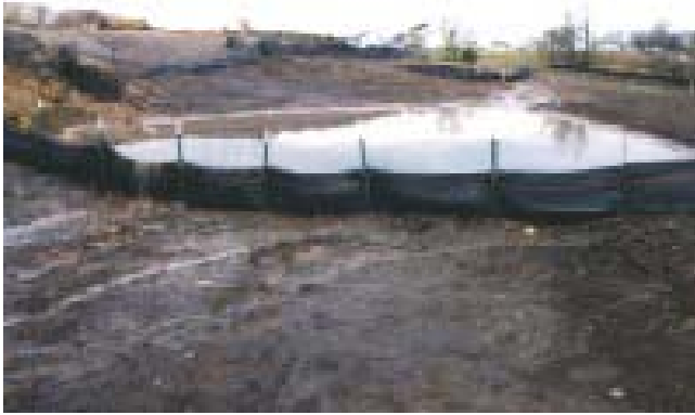
Figure 1. Properly Installed Silt Fence 1
