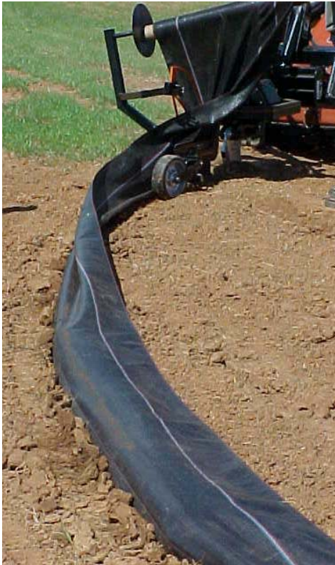
Figure 31. Curved Installation Path
