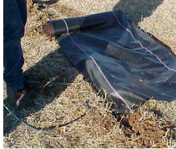
Figure 17. Silt Fence Hand-Inserted into Slot
