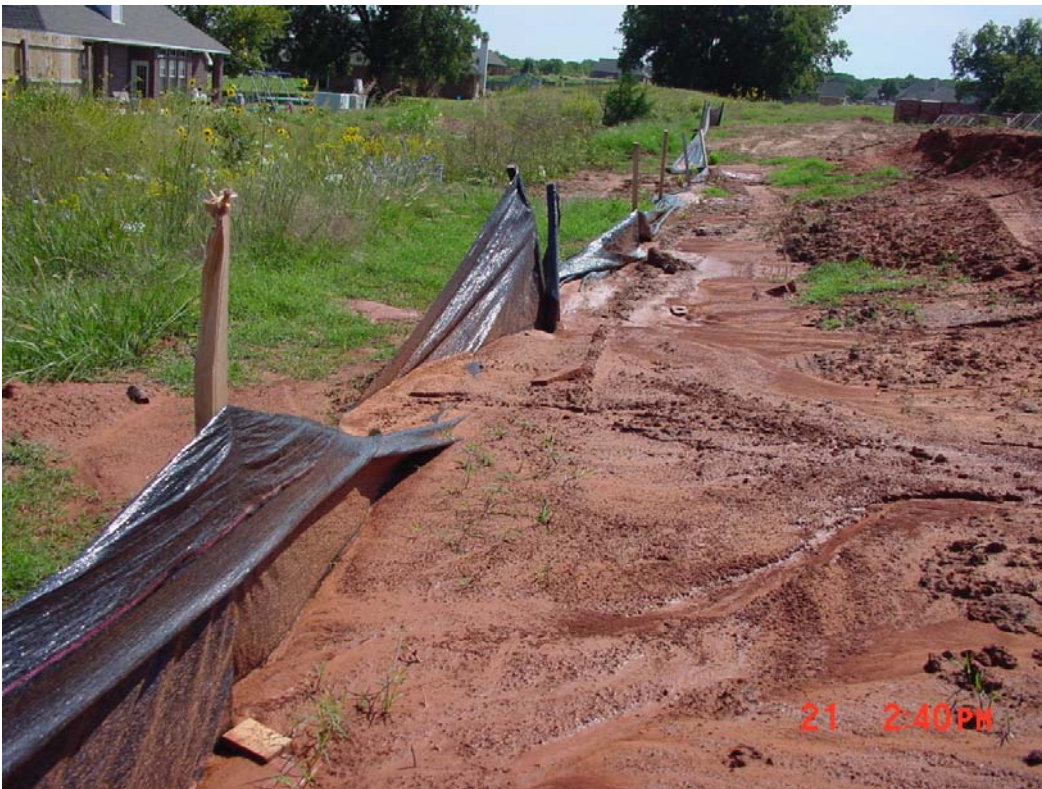
Figure 3. Failure resulting from excessive stretching and overtopping 2
