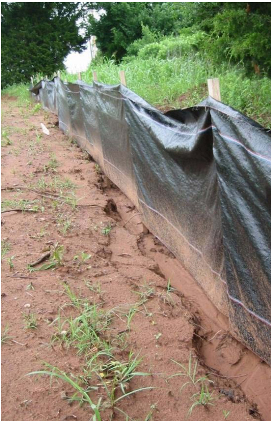
Figure 2. Failure due to Concentrated Parallel Flow (Barfield et al., 2000)
