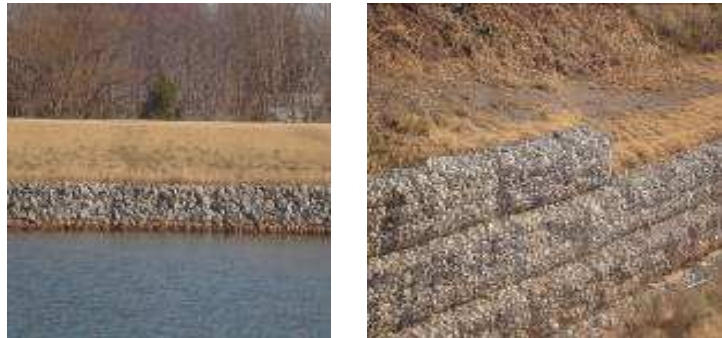
Figure 3: Rip-Rap and Rock and Gabion
