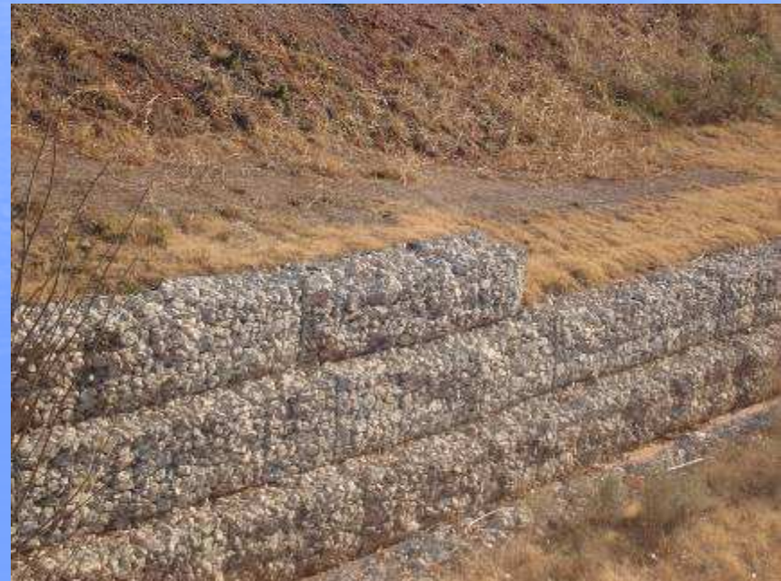
Rock and Gabion
