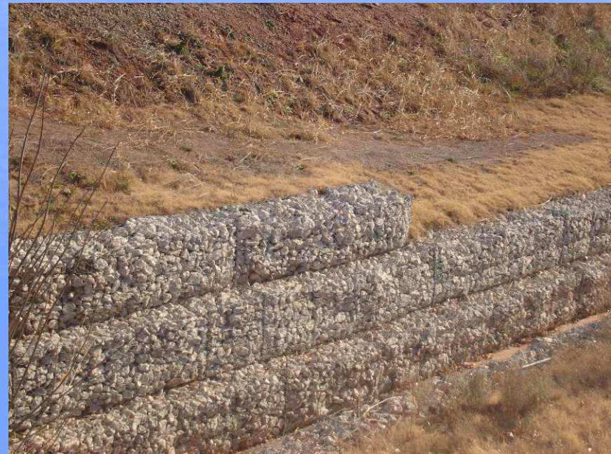
Rock and Gabion
