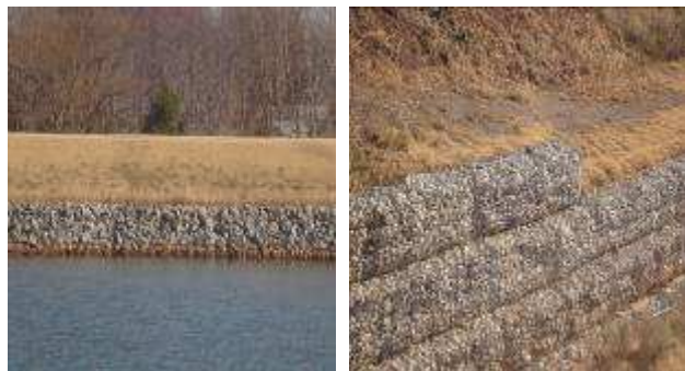
Figure 3 Rip-Rap Rock and Gabion
