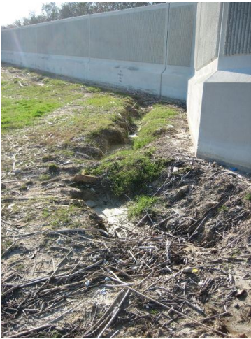
Figure 3. A floodwall scour path along the base of an existing floodwall.
