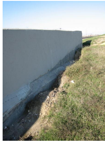
Figure 4. Floodwall scour along the base of an existing floodwall.
