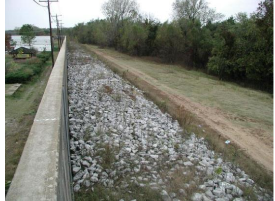
Figure 6. Floodwall with rip rap protection.
