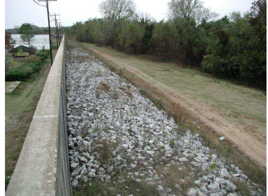
Figure 6. Floodwall with rip rap protection. (Source: http://www.uky.edu )
