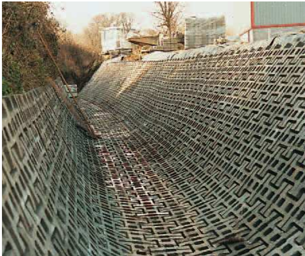
Figure 7. Armorflex® interlocking concrete.
