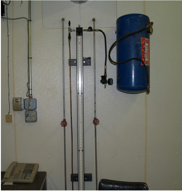
Figure 20. Manometer and air tank.
