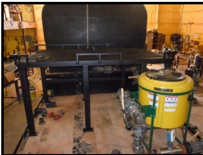
Figure 57. Elevated IBC rack to provide head pressure and space.
