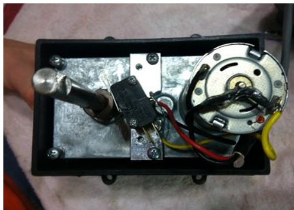
Figure 39. Repairing valves and timing cycling.
