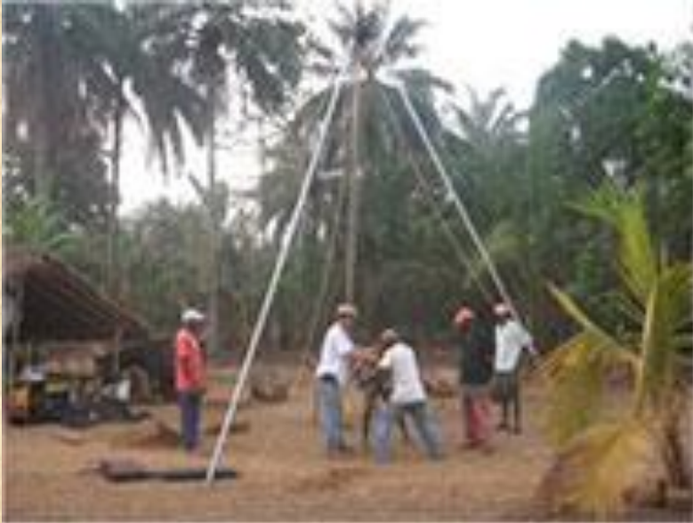
A-frame for cable tool method
