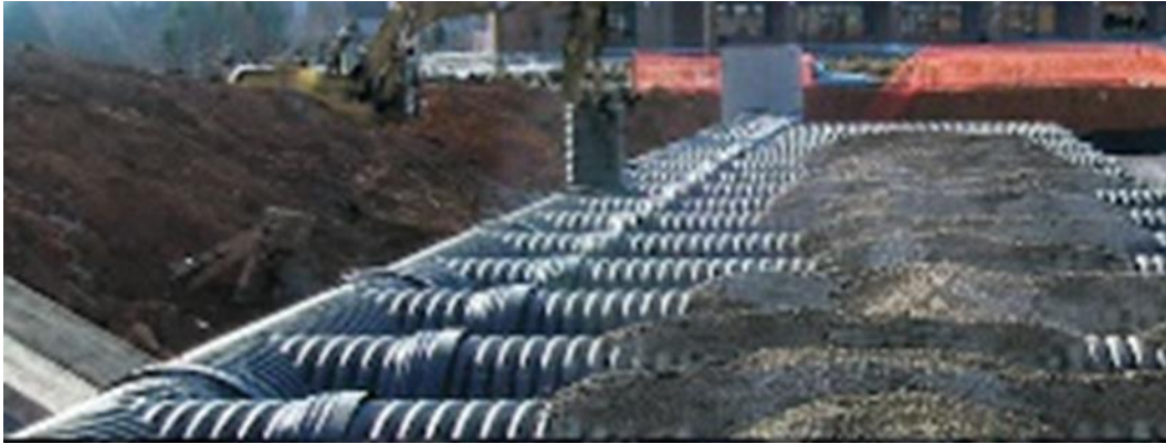
Figure 2 Construction of HDPE piping (Plastics Pipe Institute, 2014)
