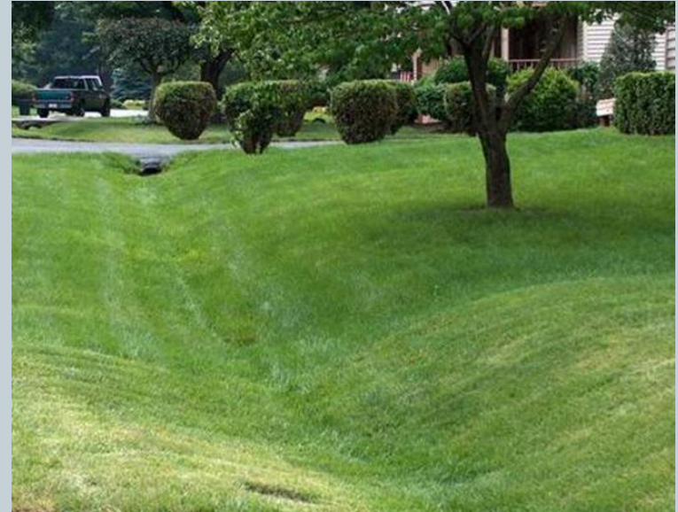
Grass-lined channel (Fairfax County, Virginia, 2014)
