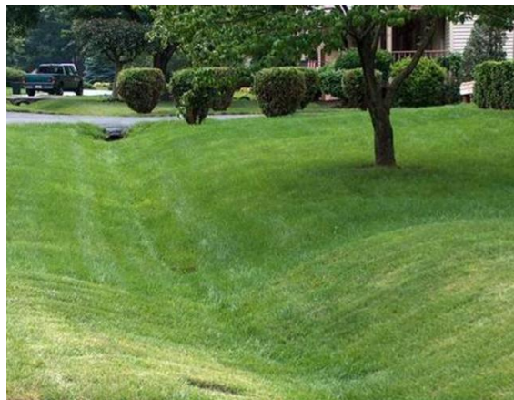
Figure H-1. Grass-lined channel illustration (Virginia DEQ, 2014)
