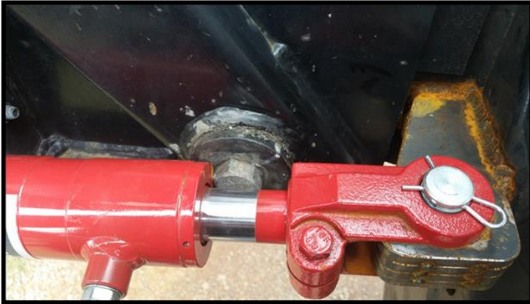
Figure 41. Cylinder Contact with Bolt Head
