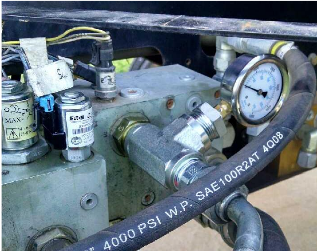
Figure 52: Pressure Gauge Plumbed into Knife Circuit
