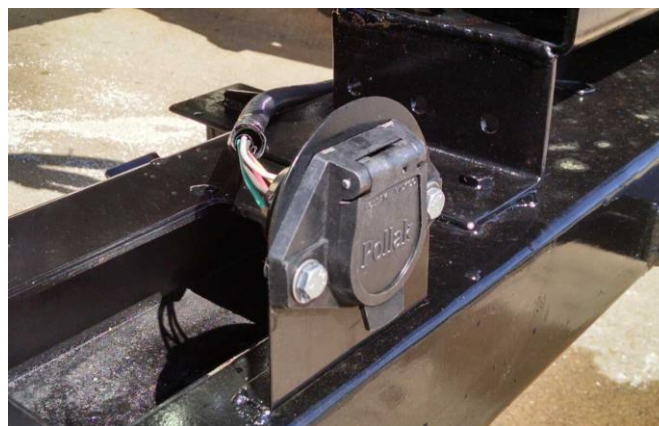
Figure 37: Trailer Wiring Connection
