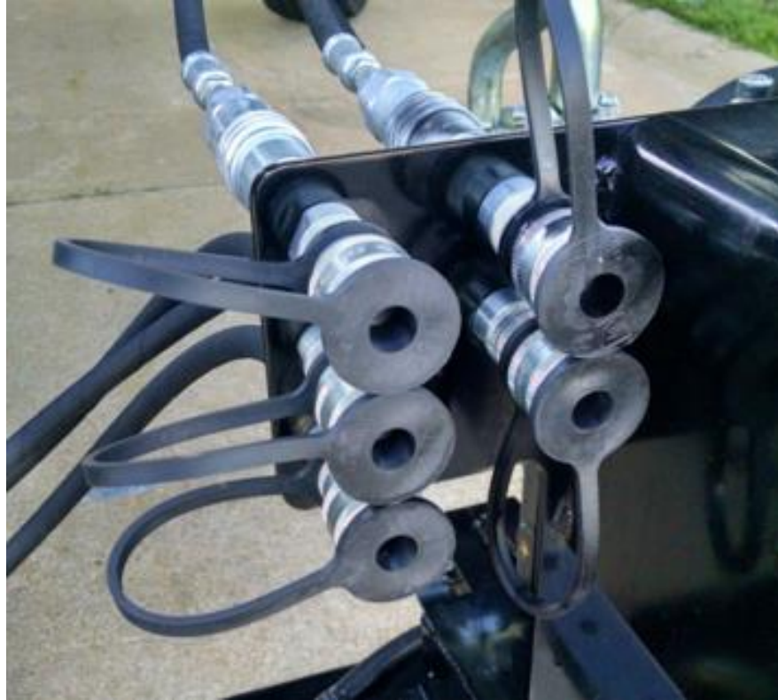
Figure 54: Hydraulic Auxiliary Outlets
