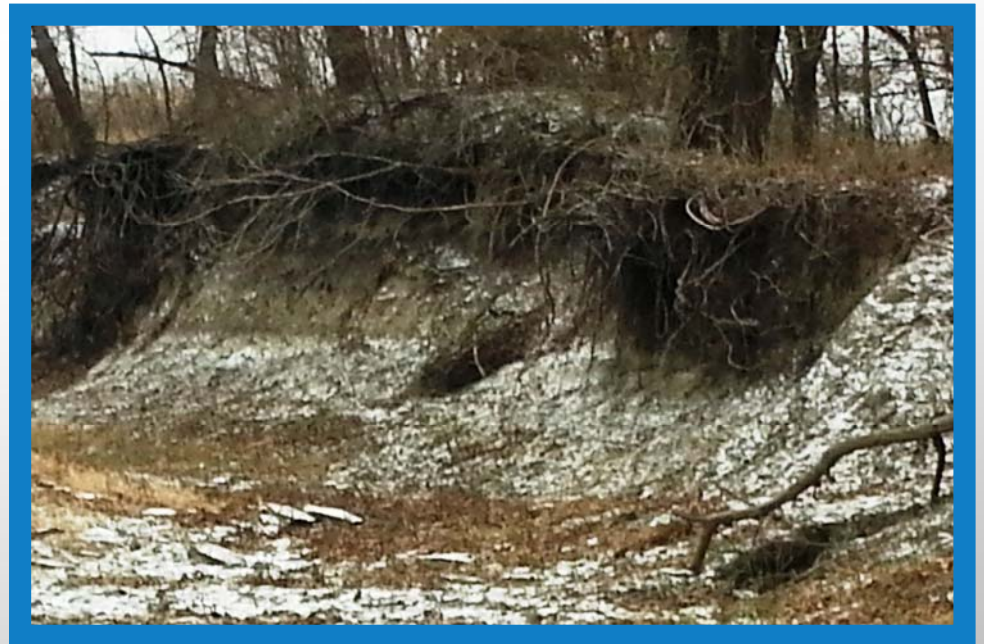
Overhanging soil held in place by roots, Site 33
