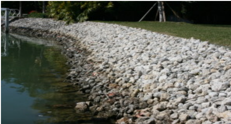
Figure D-7: Riprap along a coastal shoreline in Florida (Garland & Garland, 2014).
