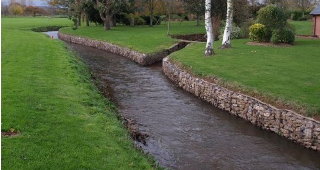
Figure 8: Gabions along an English streambank (Gabion Erosion Control, 2014).
