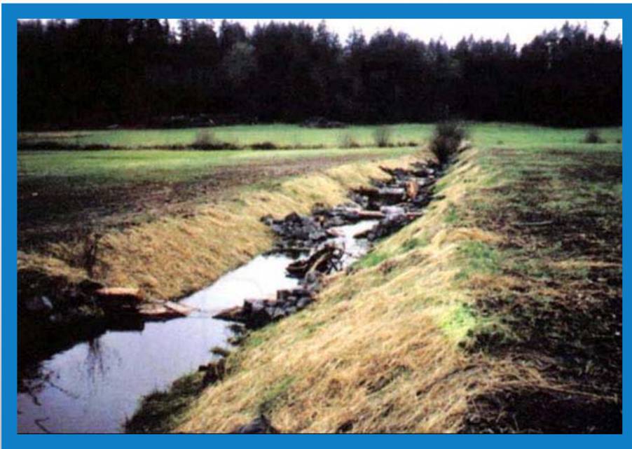
Streambank Re-grading (Washington, 2003)
