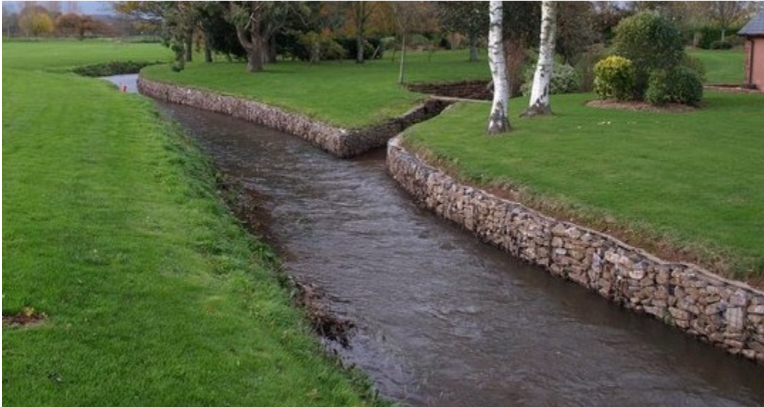
Figure D-8: Gabions along an English streambank (Gabion Erosion Control, 2014).
